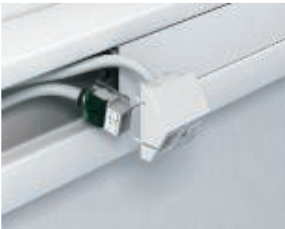
Data technology support installation – device installation Insert the complete data technology connection module into the data technology support from behind. For this, insert the support plate of the connection module into the seat and lock it in place.
